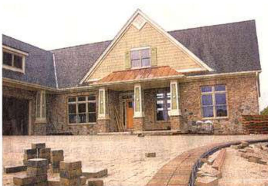
The house is covered with a mixture of brick and local stone, with a paved brick driveway.
